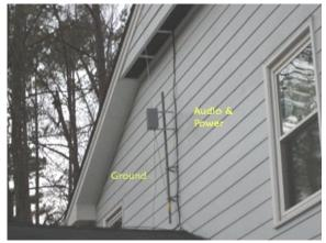
Do you see how the transmitter is mounted right next to the house? It is not above all buildings, the antenna is not in the open air, also look at the antenna, it is right up against the siding!! NO!!
